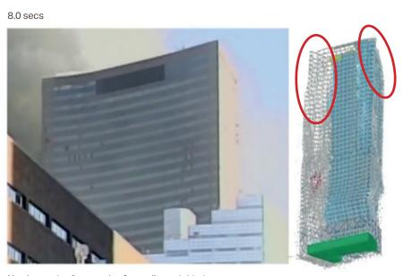
North exterior 8 seconds after collapse initiation. NIST's LS-DYNA model of the collapse.
