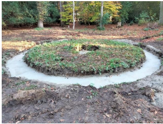
Foundations for the new turntable now in place
